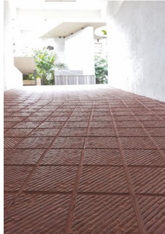
Ropeline - Basement Ramp
